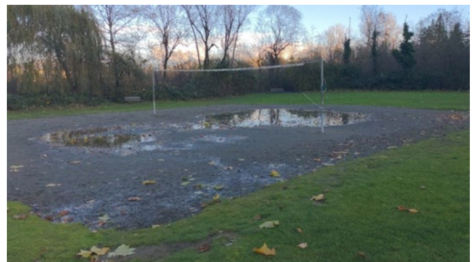
Mill Lake Park: Example of poor drainage at sand volleyball courts
