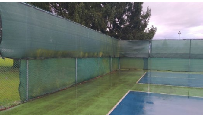
Brandner Park: Example of what is considered moderate fence condition
